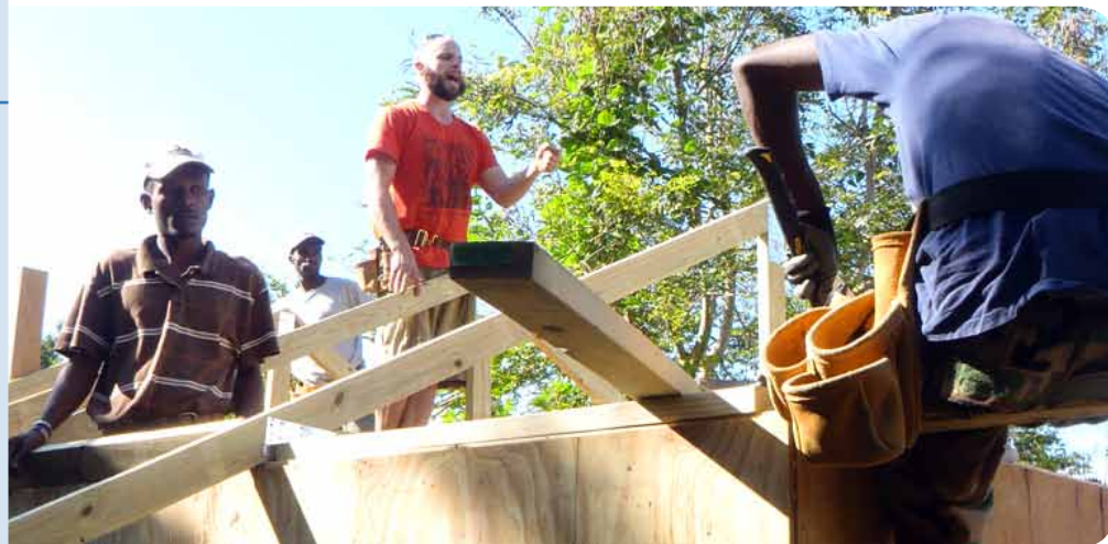
Construction of a replacement house for a Haitian family.
